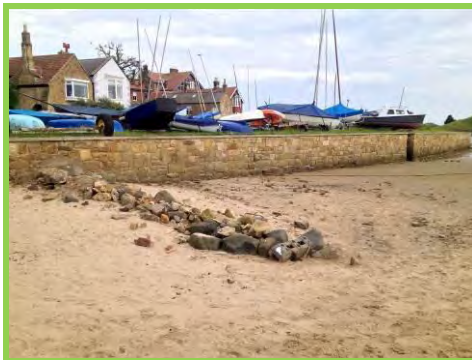
Low masonry wall at River Aln Boat Club (/2801c03).
