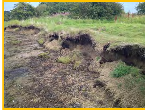
Total erosion and undermining of earth bank on upstream face of spit (2801c09).
