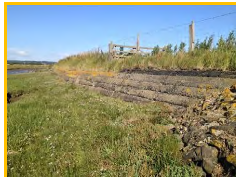
Concrete walls at Links End in fair condition (/1401c27)..
