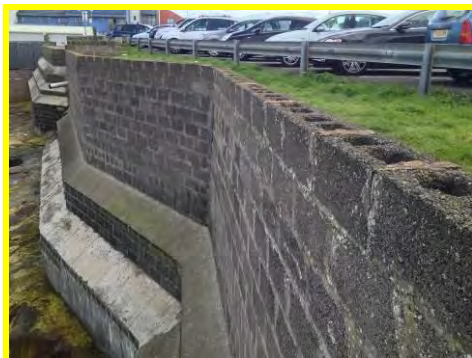
Concrete blockwork wall fronting car park in fair condition (/1701c02).
