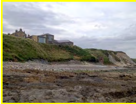
Erosion at toe of soft earth cliffs fronting Sea House (/1101c04).
