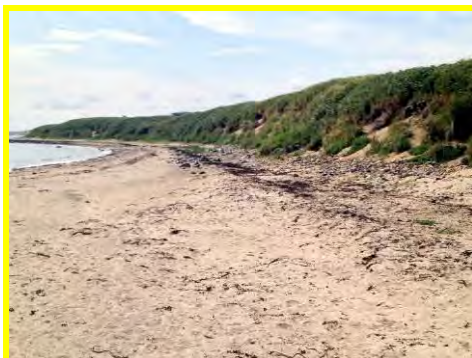
Localised erosion of low vegetated coastal slopes at Seaton Point (I2601c07).
