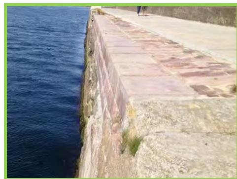
Replacement of masonry blocks and new concrete deck slab (/701c15).
