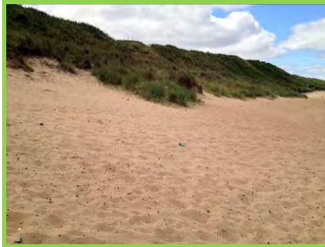
High beach levels and vegetation burying masonry wall north of harbour (/4401c01).
