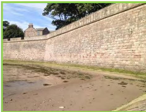
High masonry seawall wall around Fisher's Fort (/801c06).
