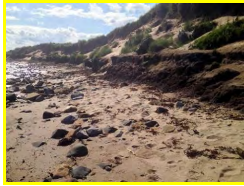
Erosion, cliffing and collapse of dunes south of Bondi Carrs (/3201c08).
