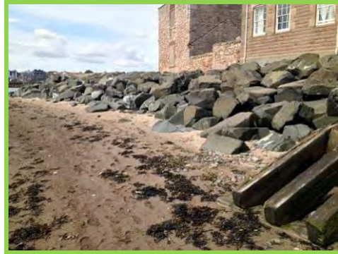
Rock revetment well packed and buried by high beach levels (/801c04).
