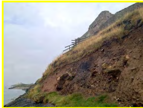
Slumps in cliff below castle east of erosion matting (/4901c12).
