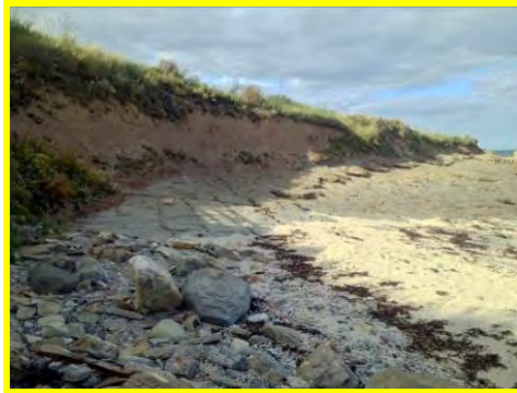
Ongoing erosion of soft cliffs south of Dell Point (/1701c30)
