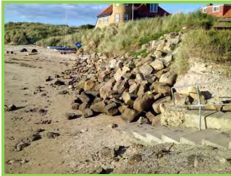
Localised dumping of rock at north end of Beadnell Bay to protect harbour road (/1701c52).
