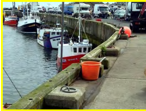
Existing quay wall at Warkworth Harbour in good condition (/3001c05).
