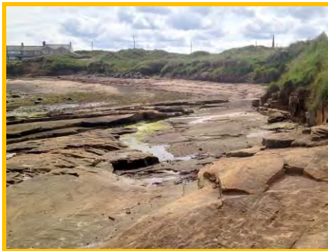
Erosion and cliffing in face of dunes along much of the Amble Links frontage (/3101c06).
