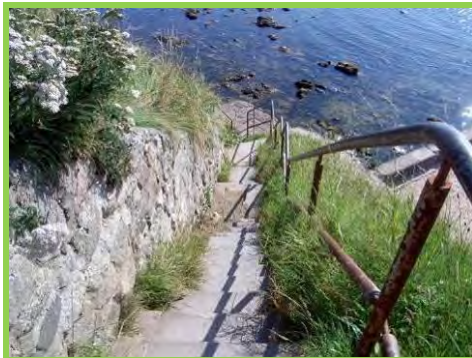
Steps and hand railing at Green's Haven in good condition (/701c05).
