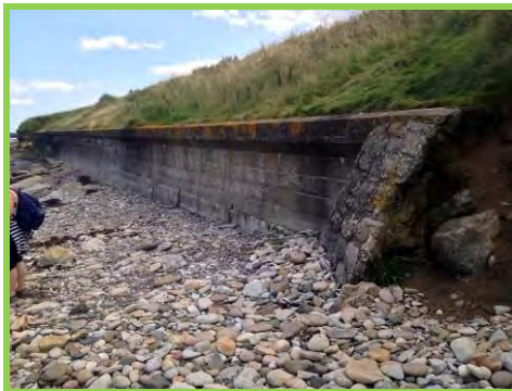
Onset of outflanking at the west end of seawall at St. Aidan's Road (/1701c54).
