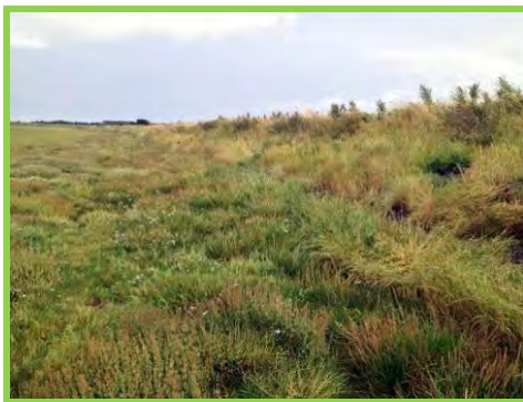
Flood embankment east of bird hide at Elwick (1401c98).
