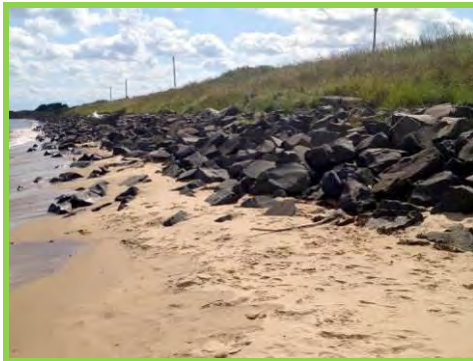
Dumped stone revetment south of Low Hauxley in good condition (/3201c03).
