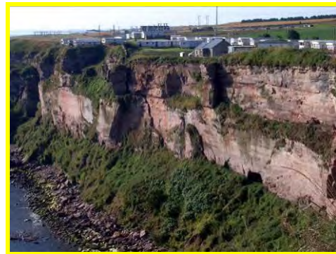
Fractures in cliffs at south end of Marshall Meadows Bay (/601c03).
