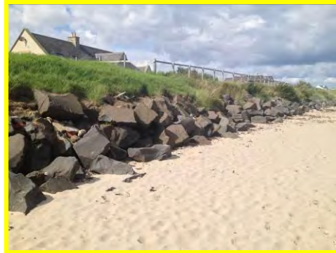
Lower beach levels fronting the rock revetment at Low Hauxley (/3201c02).
