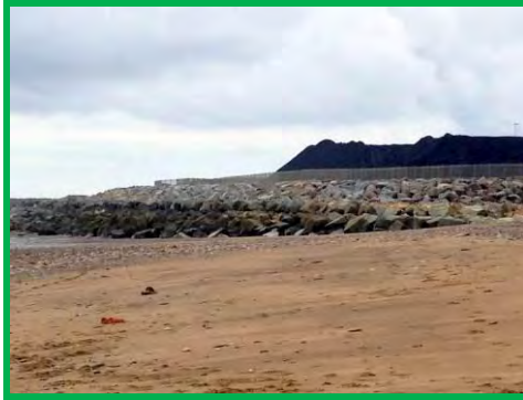
Rock armour revetment fronting coal stocking yard (/3401c07).
