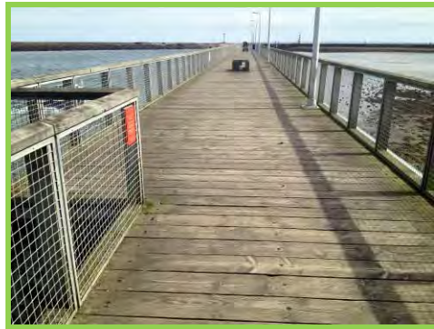
Timber decking in good condition (/3001c11).
