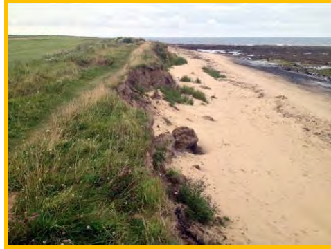
Accretion of beach material providing protection to soft cliffs in centre of bay (/3501C04).
