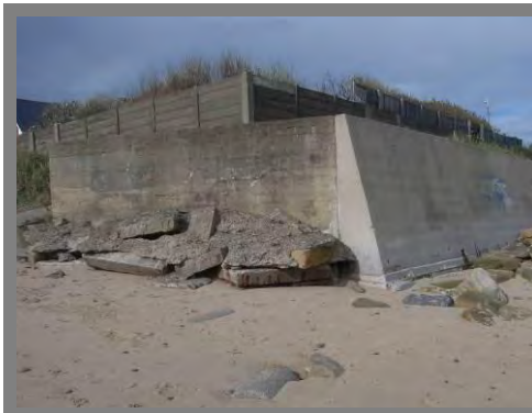
Post and plank crest wall observed in 2012.
