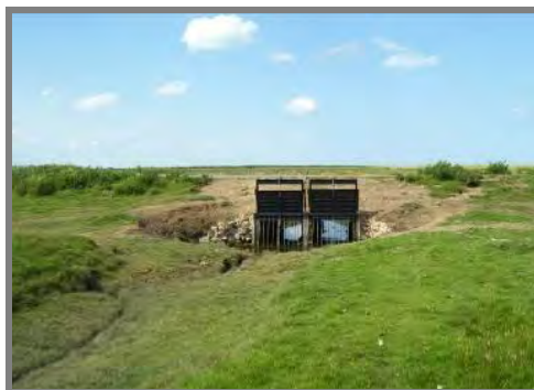
New sluice structure south of Beal Point constructed in 2010.
