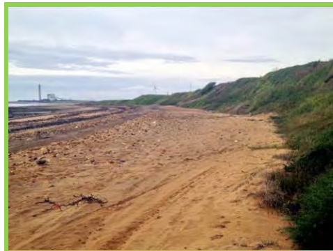
Wide spoil beach providing protection to the coastal slopes (/3401c01).
