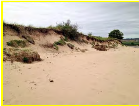
Erosion and cliffing of dunes south of Rive Aln (/2901c01).
