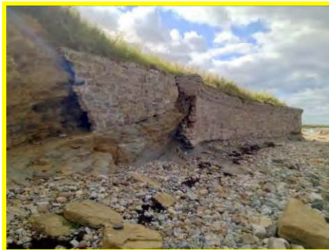
Masonry seawall north of Dell Point (/1701c25).
