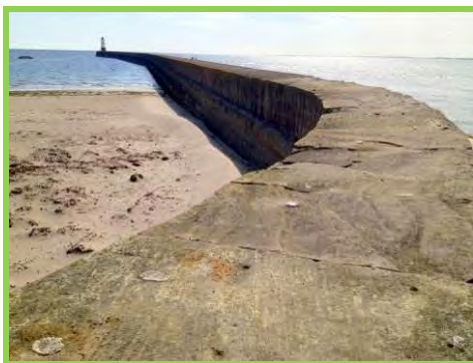
Refurbishment of the Berwick Pier completed in 2012 (/701c14).
