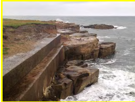
Concrete headwalls of outfall at Spital Point (/3601c10).
