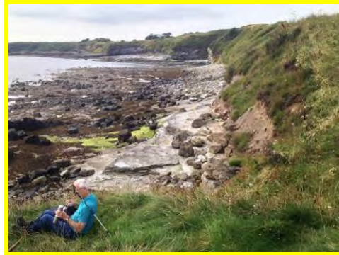
Some erosion of upper earth slopes south of Cullernose Point (2401c01).
