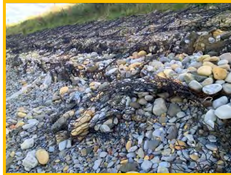
Burst baskets at the toe and loss of stone across the foreshore (/3701c39).
