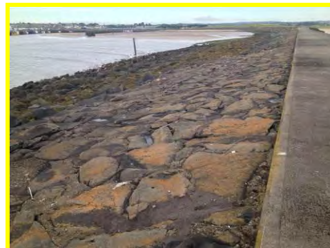
Rock armour and masonry on south face of North Pier in good condition (/3001c03).
