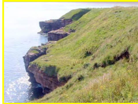
Caves and fissures in cliffs and slumps in upper soft material (/601c05).
