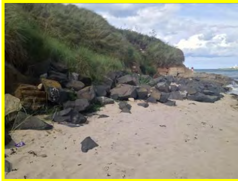
Stable vegetated cliff fronted by rock armour south of Beacon Hill (/3201c02).
