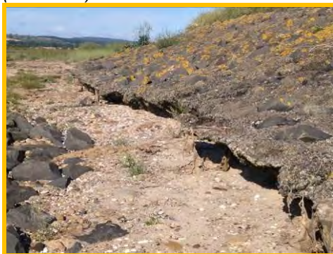
Concrete walls at Links End in fair condition (/1401c27)..
