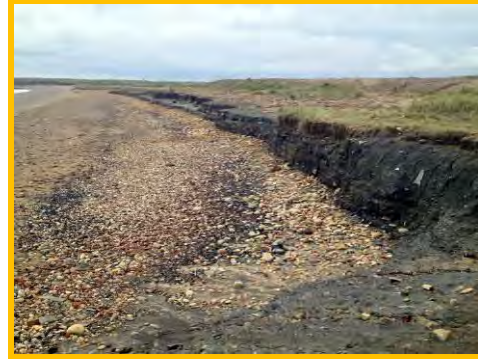
Active erosion of colliery spoil cliff at the north end of the bay (/3501C01).
