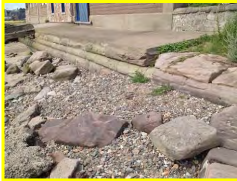
Masonry seawall buried by high beach levels (/801c05).
