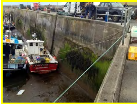
Inner concrete face of South Pier in good condition (/1701c14).
