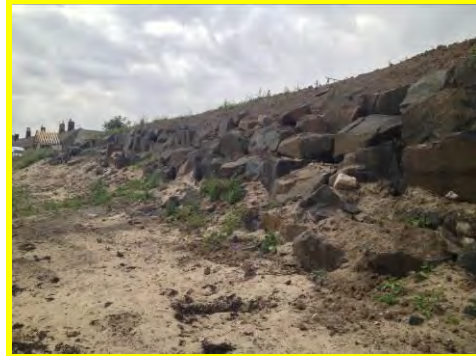
Rock armour added to south end of concrete block revetment (I2602c02).
