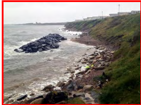
Accumulation of sand in lee of breakwaters but erosion continues (/3701c03).
