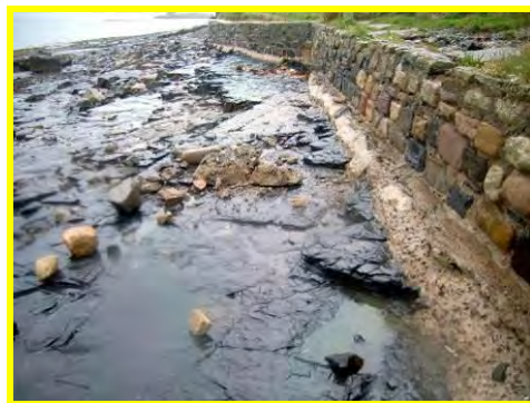
Shingle beach completely removed exposing rock foreshore in 2014 (/4901c06).
