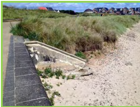
High beach levels burying the bottom of the steps south of the dunes (/4201c06).
