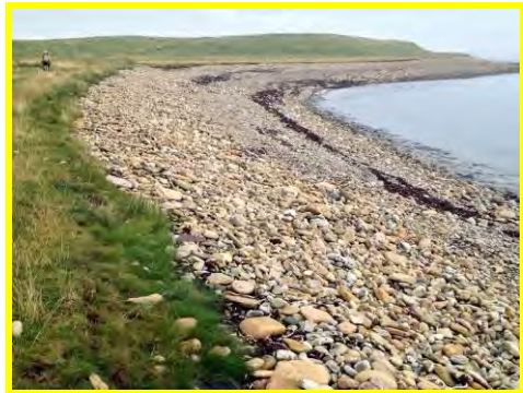
Erosion at grassed area of cobbles and shingle at Sheldrake Pool (/5001c03).
