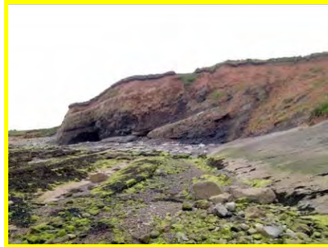
Significant but localised erosion of earth cliffs at Saltpan Rocks (1101c05).
