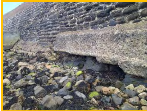
General undermining at mid-point of wall with potential loss of concrete toe works (/1701c36).
