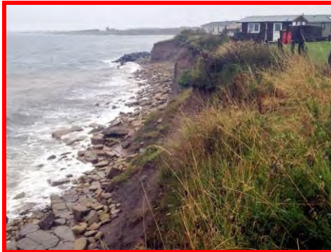
Active erosion and slumping of cliffs along the Sandy Bay Caravan park (/3701c03).
