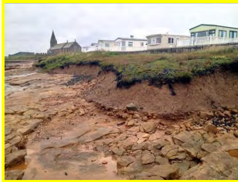
Slumps in cliffs and unravelling of soil netting west of Newbiggin Point (3601c01).
