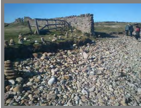
Erosion adjacent to boundary wall in 2012.
