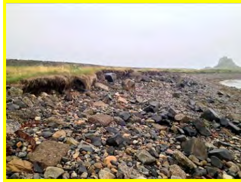
Active erosion and cliffing of earth slopes around the north side of the bay (4901c11).
