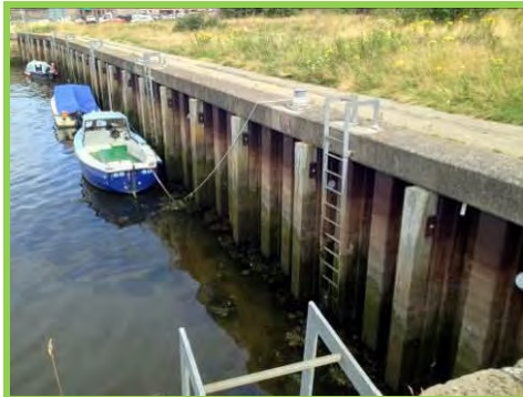
Berwick sheet piled quay wall generally in good condition (/801c03).
