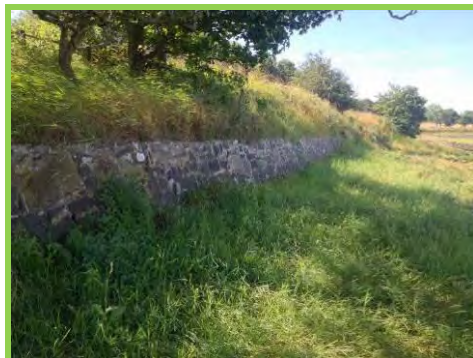
Masonry wall at south end of revetment in good condition (/1501c04).
