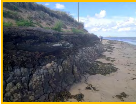
Erosion of lower peat layer and cliffing in the upper slopes south of Bondi Carrs (/3201c07).
