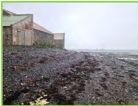
Increase in crest level of the shingle beach in front of boat houses (/4901c05).
