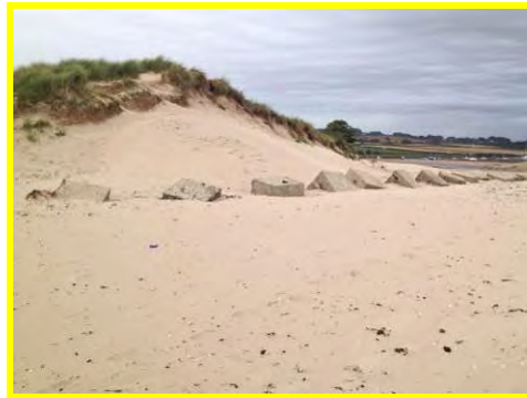
Cutting back of dunes south of River Aln despite the presence of concrete blocks (/2901c01).
