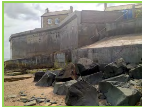
Seawall at Wellhaugh Point in good condition (/3101c07).
