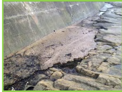
New sealant to joints in recurved seawall (/3601c13).
