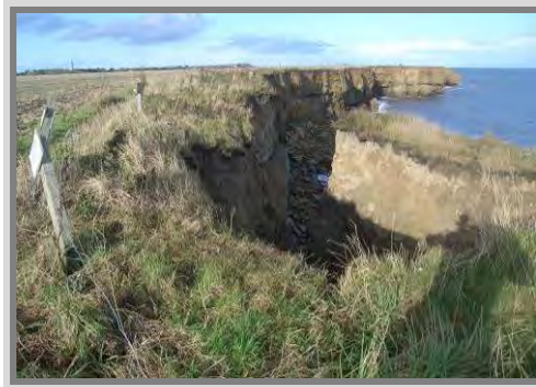
Partially collapsed cliff and closed footpath at Hawk Cliffs. In 2012.
