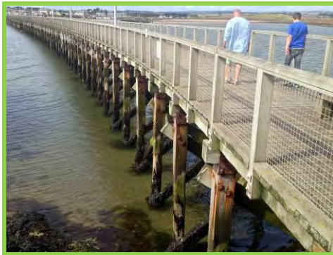
Timber piles and superstructure of South Jetty in good condition (/3001c11).
