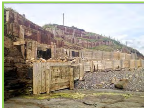
Timber breastwork extended in 2010 to prevent slips in upper slopes (/3301c01).
