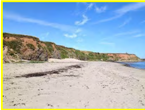
Slump in soft upper cliffs at Bucket Rocks (/701c12).
