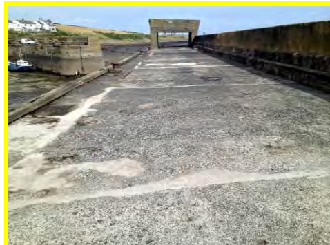
Recent repairs to the concrete decking on the south pier (/2201c11).
