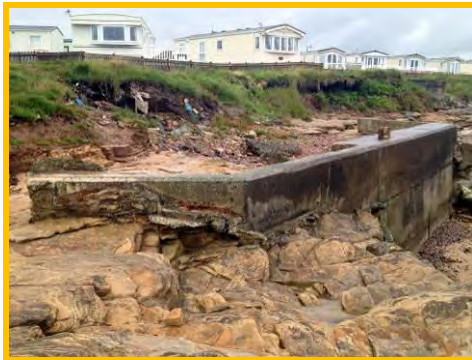
Outflanking and erosion behind the crest of the concrete wall at Newbiggin Point (/3501C08).
