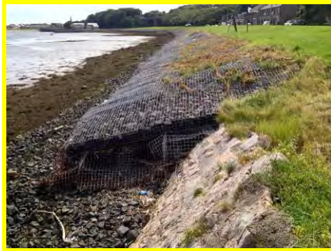
Gabion structure providing erosion protection along Dock Road (/901c04).
