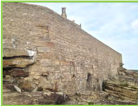
High masonry wall around The Bathing House in good condition (/2401c02).
