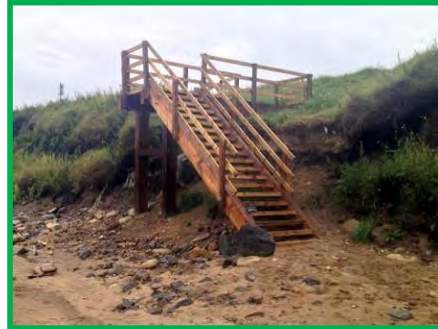
New timber stairs constructed adjacent to southern car park (/3901c03).
