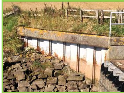
Sheet piles at the sluice repainted in 2008 (/1401c19).
