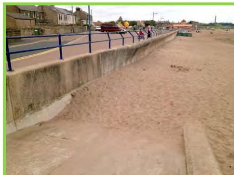
High beach levels up to underside of recurve in many places (/1001c02).
