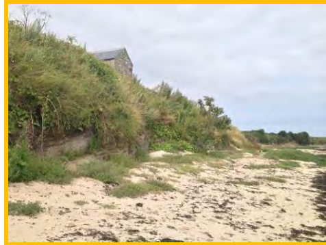
Property within a few metres of cliff edge at Boulmer (I2601c01).
