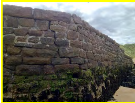
Vertical crack and missing block at seaward end of east harbour wall (/4401c03).
