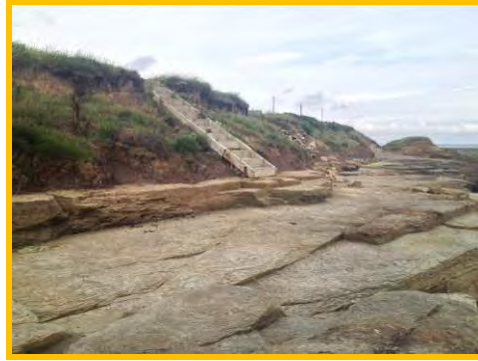
No recession evident in earth cliffs behind access steps at Snab Point (/3301c01).
