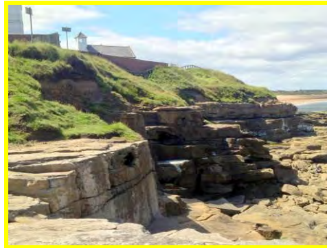
Slumps in the upper soft material cutting back to the footpath (/4401c12).
