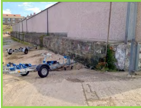
Masonry wall along back of sheds in good condition (/1701c15).
