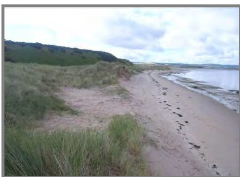
Erosion at toe of dunes fronting Heather Cottages in 2012.
