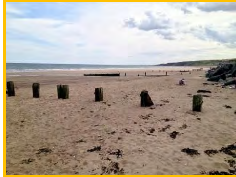
Groyne at Sandstell Point almost completely buried (/901C10).
