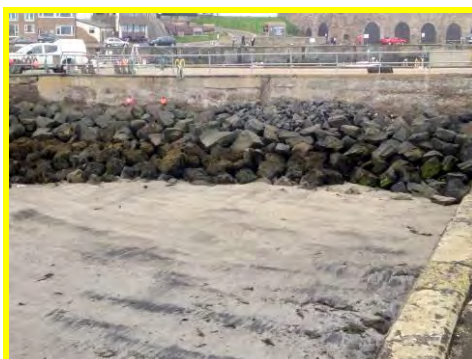
Rock armour attenuation with smaller rocks along crest (/1701c10).
