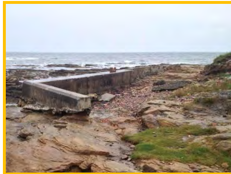
Outflanking and erosion behind the crest of the concrete wall at Newbiggin Point (/3501C08).
