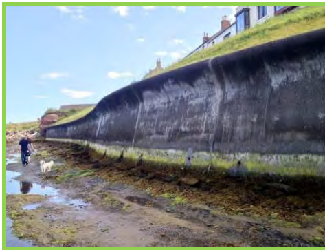
Concrete Seawall south of North Sunderland Harbour in good condition (/1701c18).
