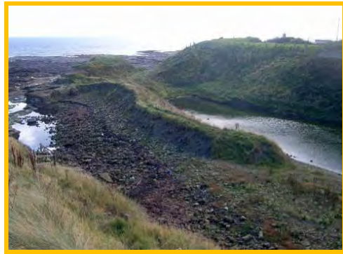
Erosion along the mound of land at the disused quarry has not worsened (/3301c01).
