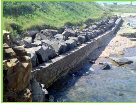
Low masonry wall at Wellhaugh Point in good condition (/3101c10).
