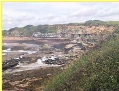
Rock falls and erosion of the soft upper cliffs at the north end of Lynemouth Bay (/3301c02).
