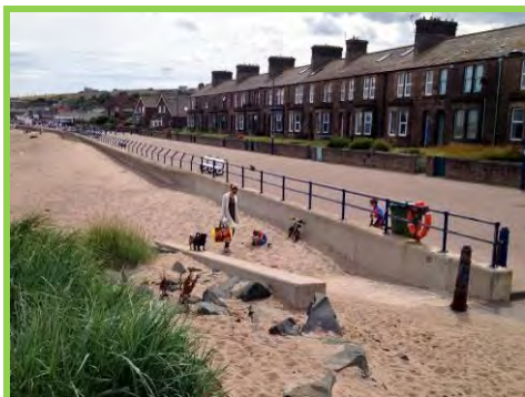
Spittal seawall, hand railing and surfacing in good condition (/1001c02).
