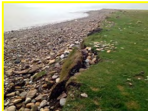
Erosion and undermining of grassed shingle on north side of ness (4901c14).
