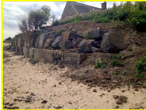
Rock armour added to north end of concrete block revetment (I2602c02).
